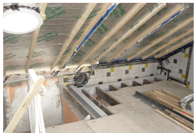
Insulation & repairs at 9 St Vincent Street
