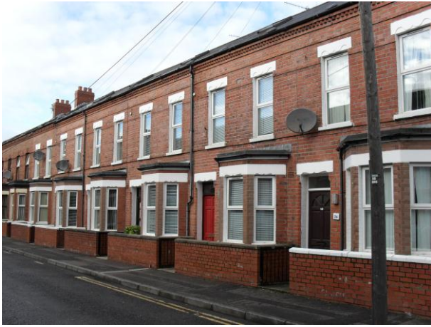
St Aubyn Street
