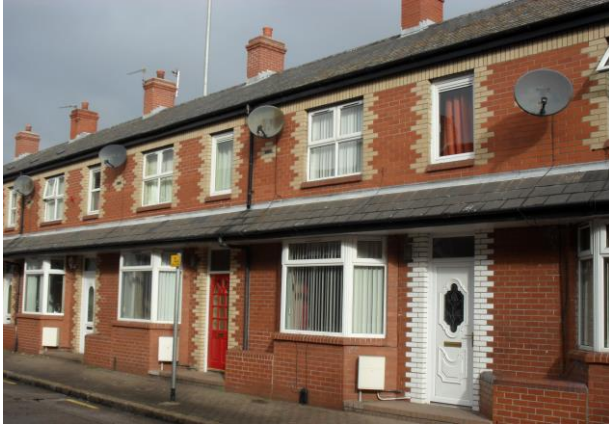
St Vincent Street – built in 1983 and an early example of new houses using traditional Belfast brick patterns
