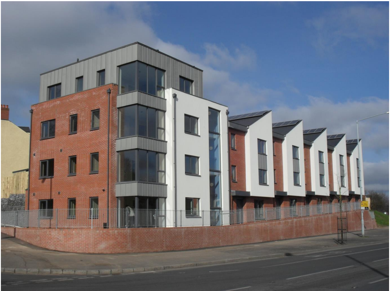
Loughview Terrace development on completion, February 2013
