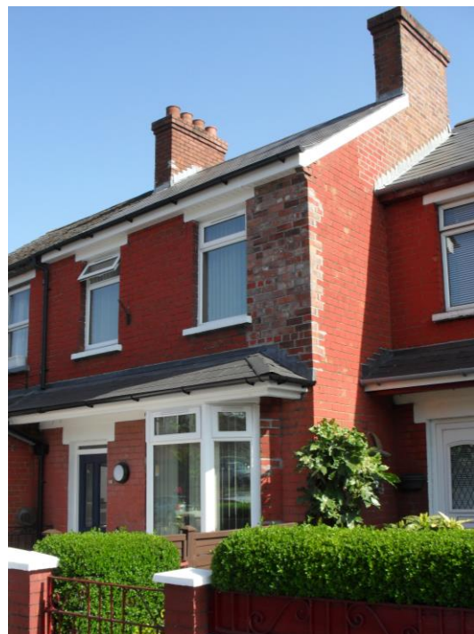
163 York Road - derelict for many years until rehabilitated in 2012
